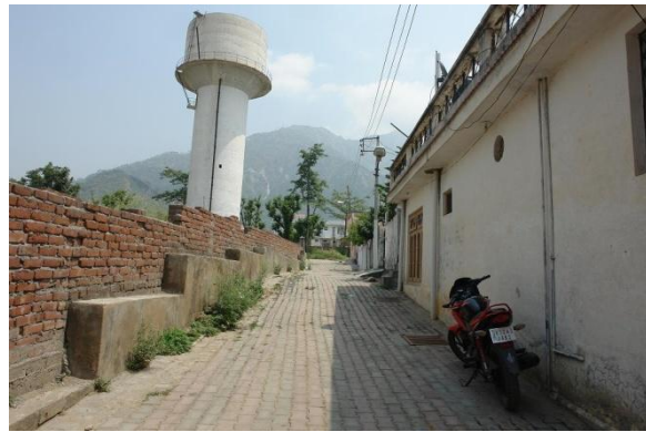
Picture 5-1: Overhead water tank
